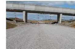
6F8 for sub-grade filling
