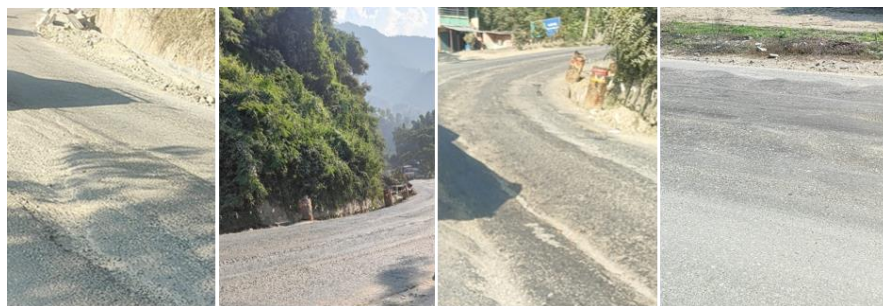
Figure 2: Rutted and depressed road surfaces in the heavily loaded truck lane of Prithvi Highway: Piplamod, Kathmandu (First Figure), Galchhi Height, Dhading (Second Figure), Richoktar, Malekhu, Dhading (Third Figure), and Bishaltar, Chitwan (Fourth Figure)
